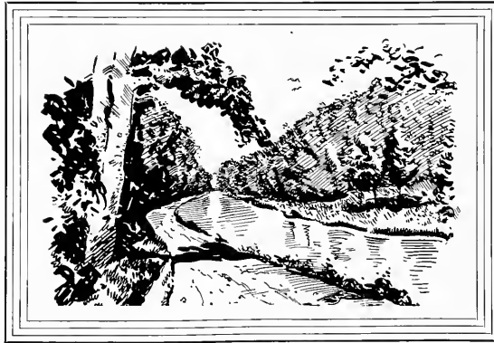
The Canal, the Towpath, and Butler's "Old Iron Bridge"
